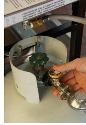
13. Using the soapy water solution provided, pour a small amount on the connections either side of the gas safety valve.
